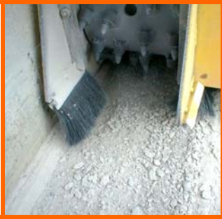
Randnahes Arbeiten / Working close to the rim
